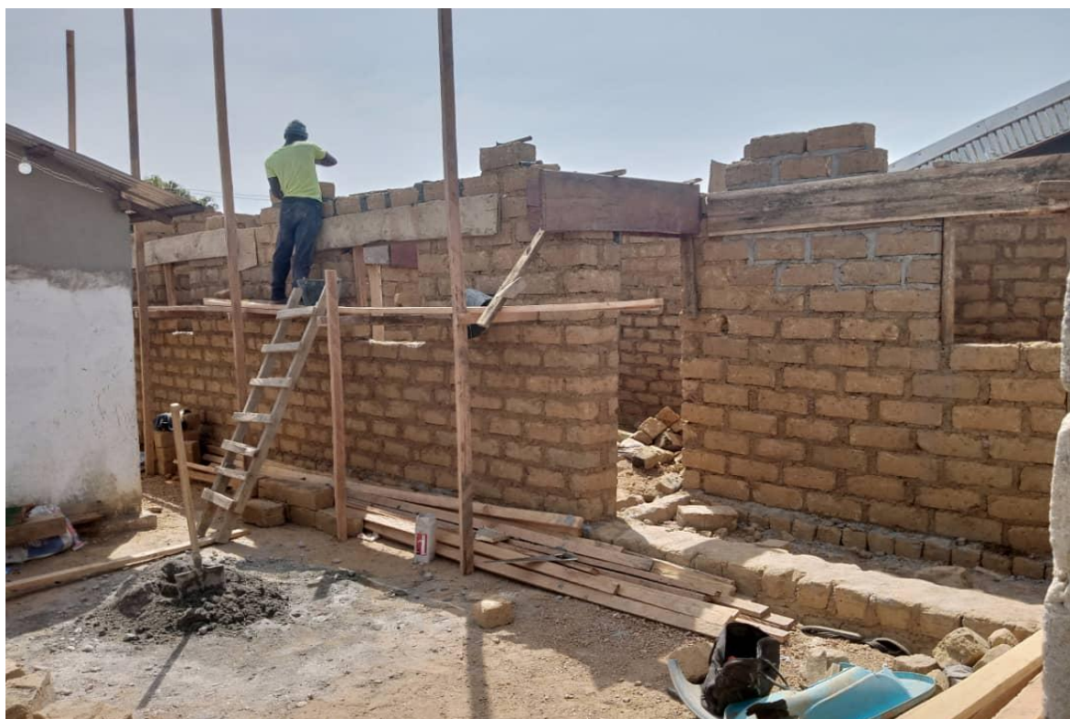
Photo 8: Chantier de construction.
