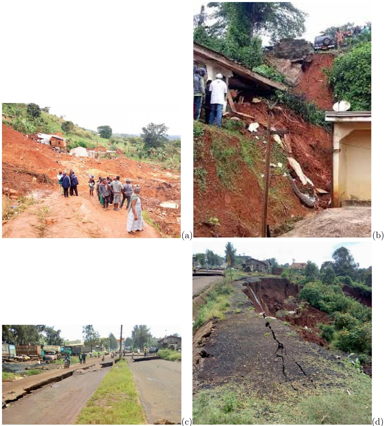
**Figure 1.8:** *Examples of traffic disruption due to key network component failures: (a) The landslide at Gouache, Bafoussam. (b) landslide at Gouache (c) In Bafoussam, in western Cameroon, a landslide in early November caused large cracks on a tarmac track; (d) The erosion has washed away part of the sidewalk from the track.*
