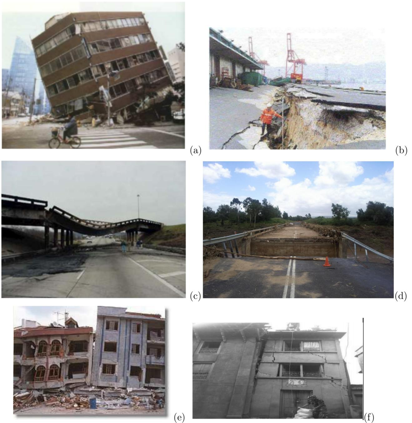
**Figure 1.7:** *Examples of the Kobe earthquake aftermath. Picture on the right shows damage: Partial collapse or total collapse of civil structures caused by liquefaction: (a) building, (b) landslides/creep (c) bridges/tunnel, (d)scupper-hole, (e) Building pounding (New Zealand 2009) [11], (f) Pounding effect between two buildings [43]*
