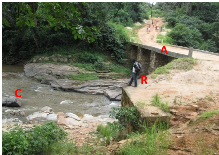
Photo 5: Bridge over River Mafup in Kom (Mfumte)
