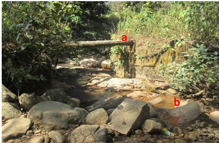
Photo 4: An unbridged stream with a tree trunk placed over it
