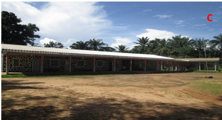
Photo A: The St Kizito Health Center, Mbaw
