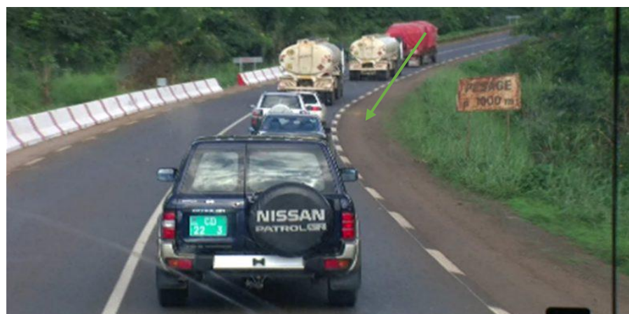
Photo 8 : Bameda-Mamfe highway and weathered road signs
