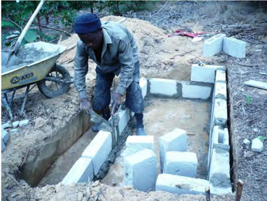
Photo 17: Construction de la cuve (A) (Cliché Mayima, 2011)
