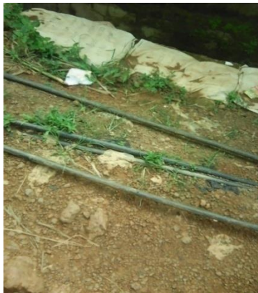
(a) Exposed pipes, (b) Pipe broken because of digging (c) Pipe broken by car exposed.
