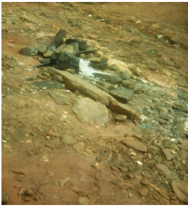
(a) Exposed pipes, (b) Pipe broken because of digging (c) Pipe broken by car exposed.
