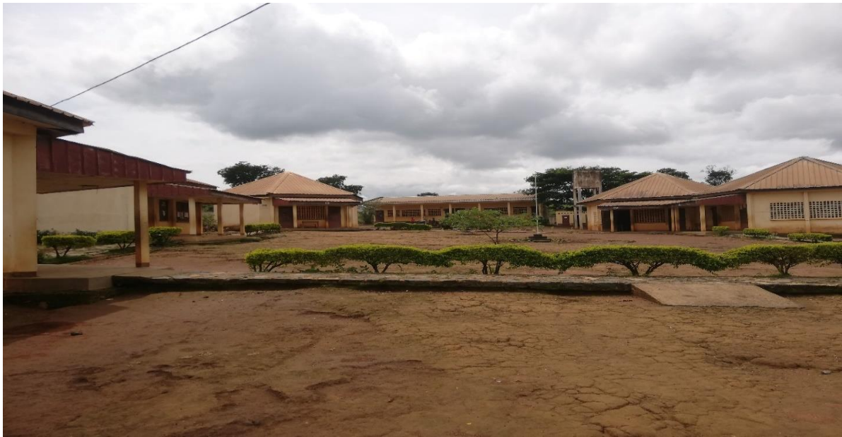
Plate 1: A partial view of School constructed by IsDBG in Gbakoungue 2000
