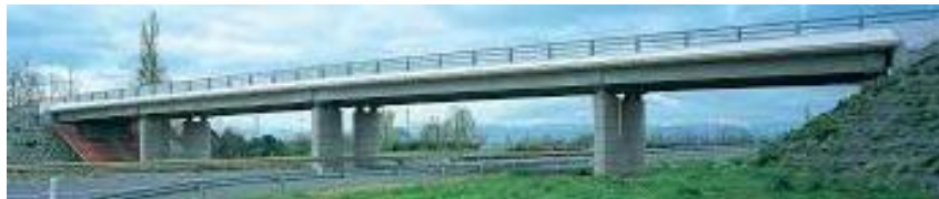
Figure 3.14: Real model of the structure
