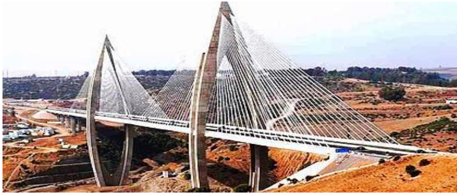
Figure 3.1: Real model of the structure (Pont Mohammed VI à Rabat).
