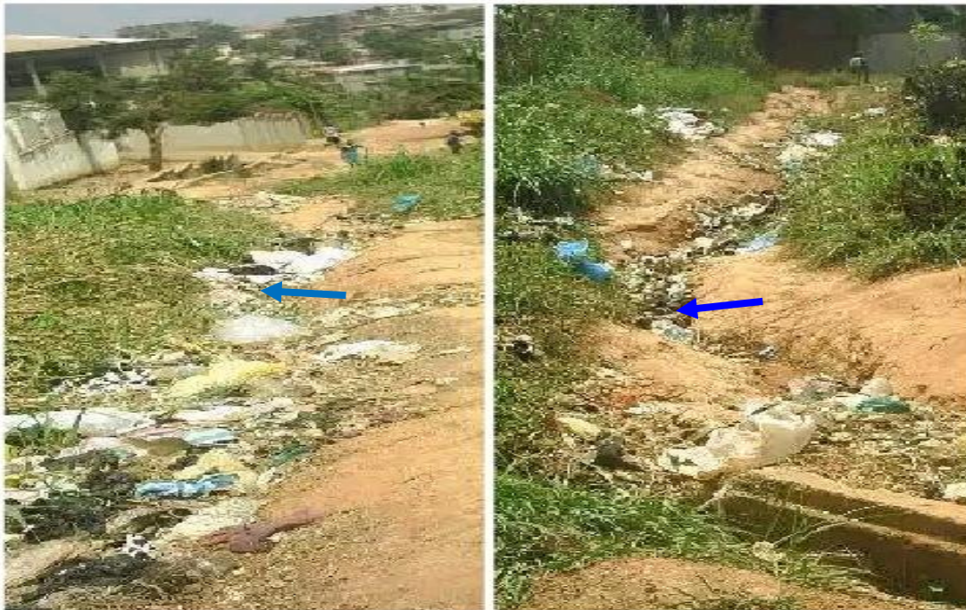
Plate 15: Inaccessible nature of the road
