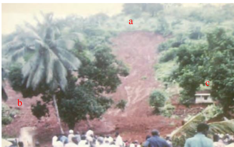
Photo 7: The Mabeta new lay out landslide of June 2001.
