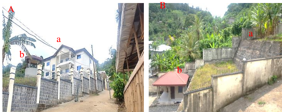
Plate 7 : Retaining wall at Bonjo Source: photo by Eti, November 2020
