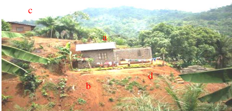
Photo 9: Anarchical construction at Mabeta new lay out.
