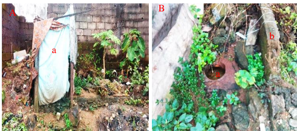
Plate 6: photos showing a pit toilet at lower Mawoh
