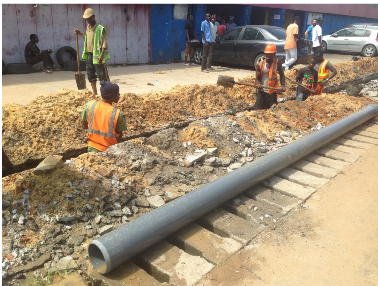
Pose de tubes SOTICI PVC Pression 315 PN16 – ABIDJAN / CI
