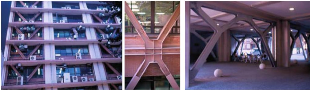
Figure 1.18. Exemple de contreventement métallique (University of Tokyo buildings) (Fardis 2009)
