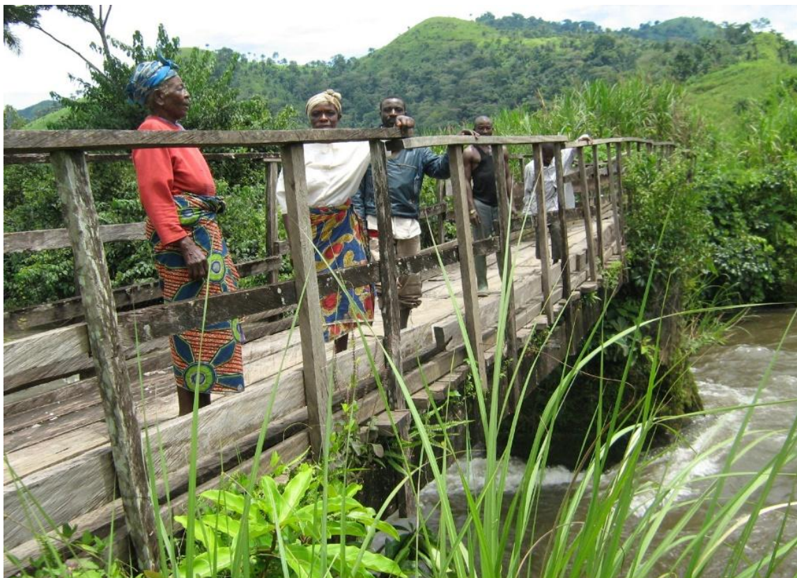
Plate 9: Bridge constructed by WADA,1982
