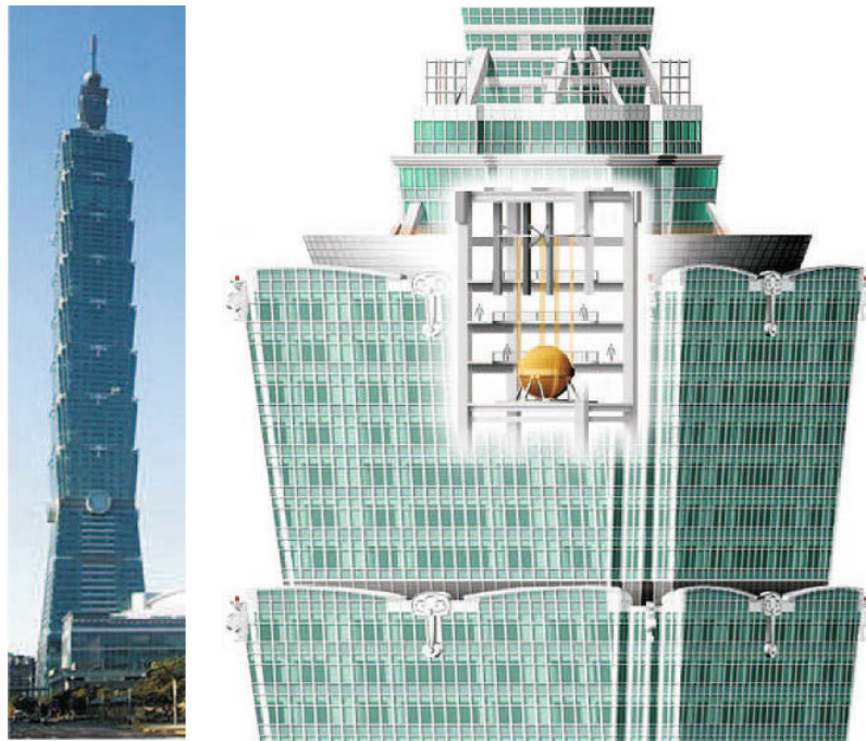
FIGURE 5 – Dynamic Vibration Absorber (DVA) of the Taipei 101 building. The DVA consists of a pendulum with a mass of 730 tons suspended with 4 cables extending over 4 floors.
