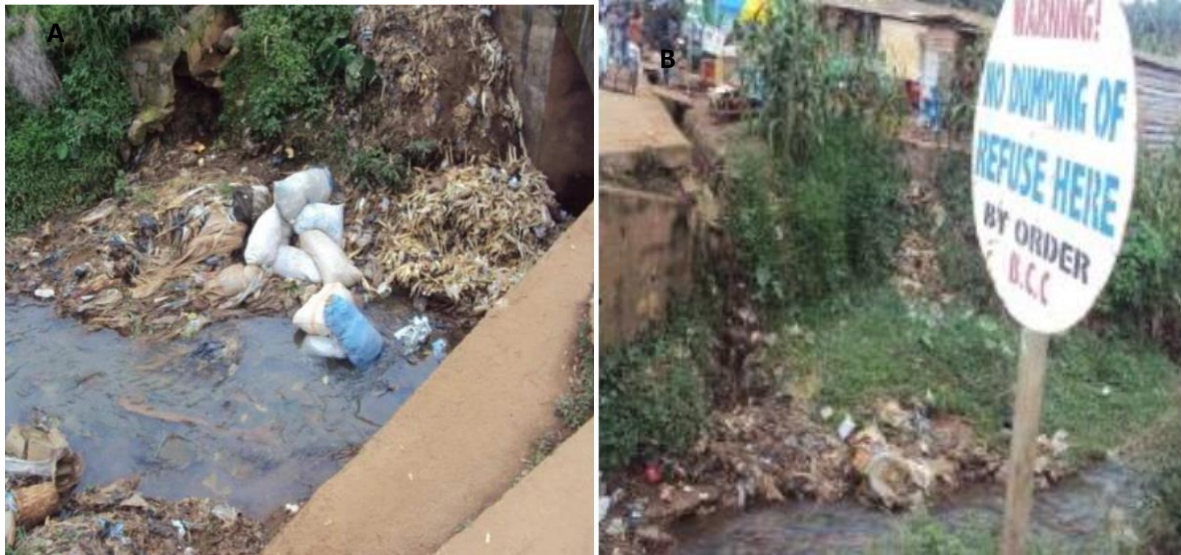
Figure 2: Dumping of domestic waste into river channel ( Source: Fogwe, 2016).
